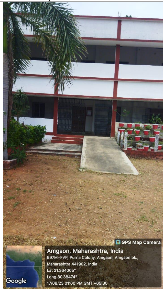
Ramp for disabled Students
